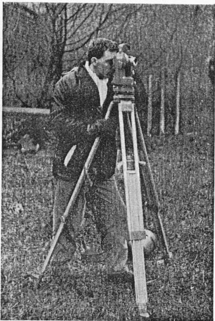
Surveying the site using a theodolite
