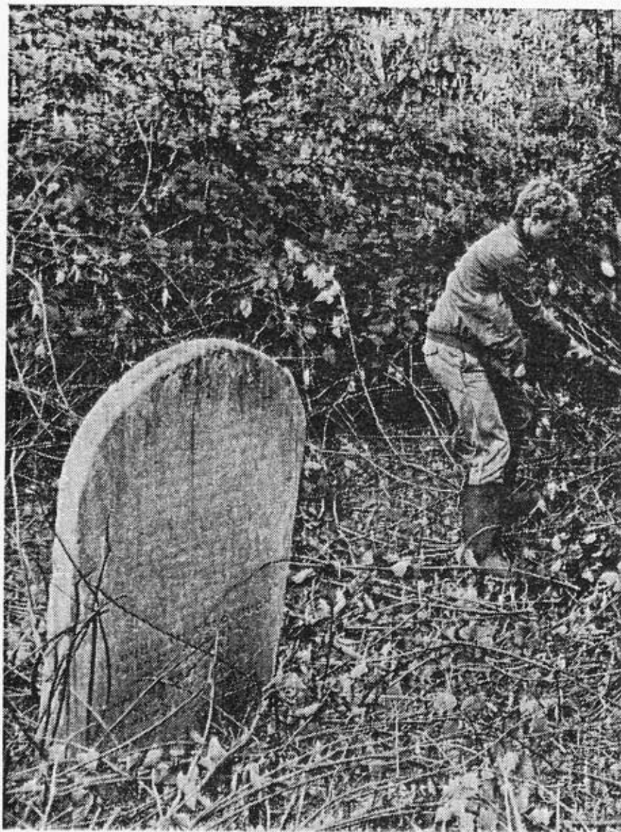
Clearing the site using a weed-eater, October 1987 (photograph courtesy of Irish Times)
