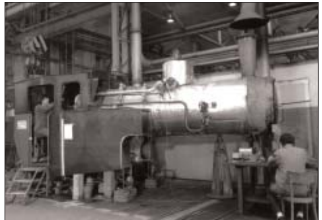
Fig. 2: Test stand for the new light oil firing. The boiler is provisionally insulated. The cab is a mock-up.
